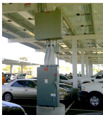
Column Mounted Equipment
