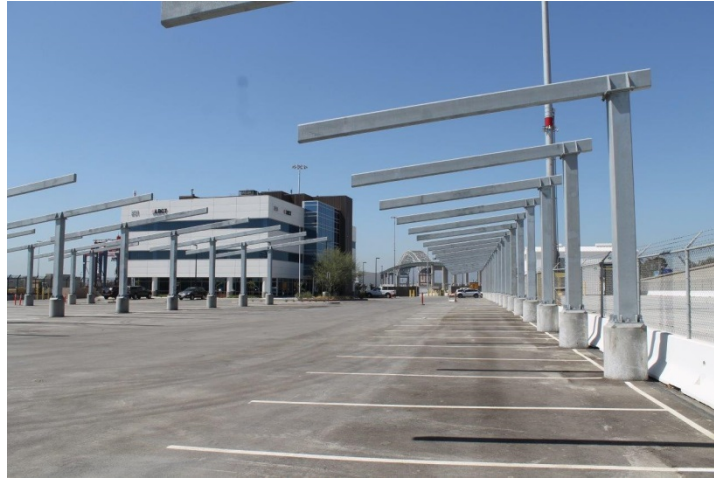
Cantilevered Gantry/Canopy Structure
