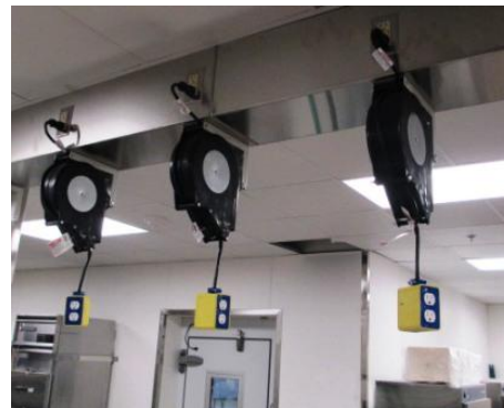
Power Cable Reel
