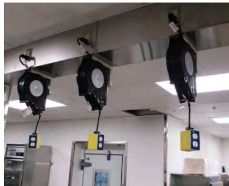
Power Cable Reel
