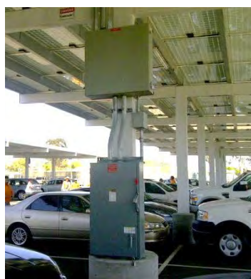
Column Mounted Equipment
